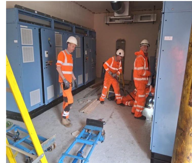
Installation of the Motor Control Centre electrical components
