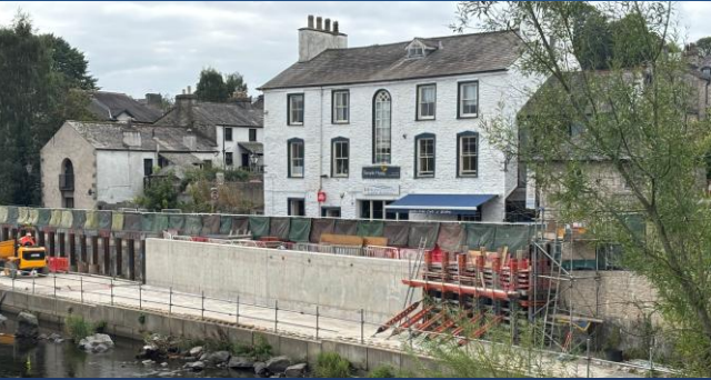
Construction of the flood wall at Waterside
