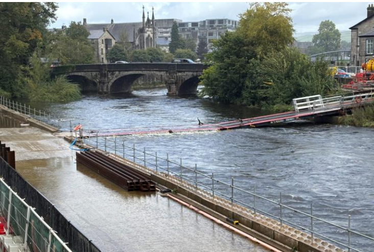
Temporary bridge at Waterside unpassable for the machinery following heavy rainfall
