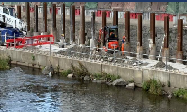
Inserting of king posts at Waterside
