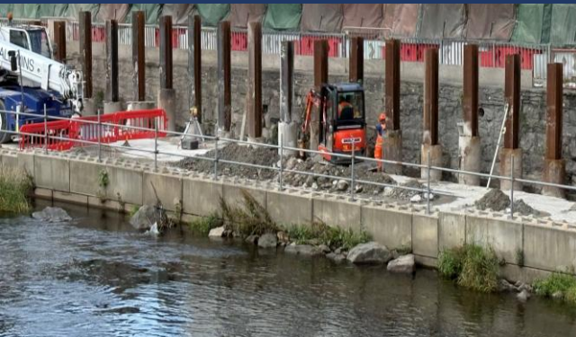
Inserting of king posts at Waterside
