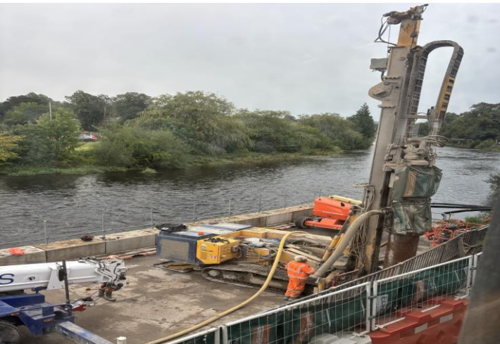
Piling towards the end of the platform at Edgecombe Court
