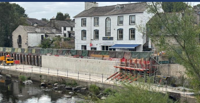
Construction of the flood wall at Waterside
