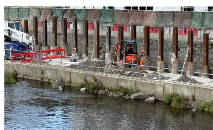
Inserting of king posts at Waterside to continue down stream
