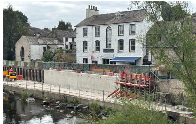
Construction of the flood wall at Waterside
