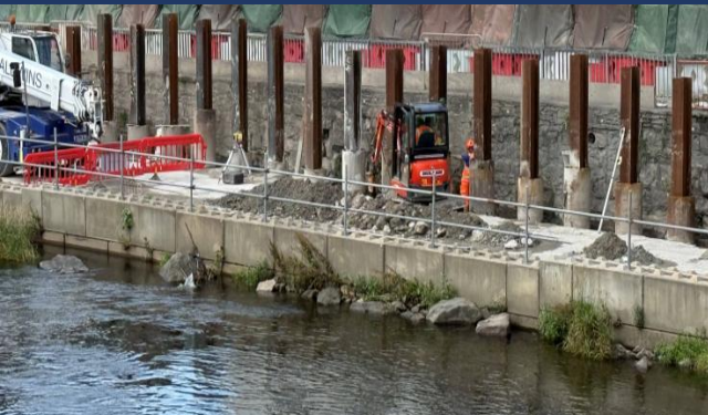
Inserting of king posts at Waterside
