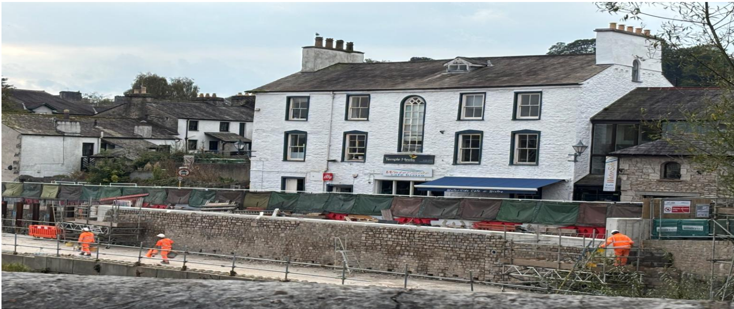
Waterside working platform showing the new concrete flood defence wall ready to be cladded – the king posts being inserted down stream
