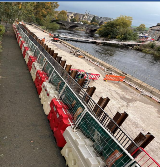
Working Platform view from Edgecombe Court
