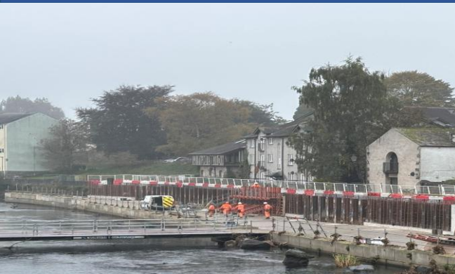
Working Platform view from Edgecombe Court
