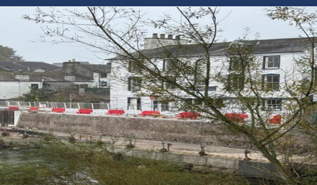
Cladded wall at Riverside Cafe
