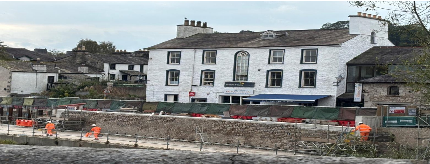
Waterside working platform showing the new concrete flood defence wall ready to be cladded – the king posts being inserted down stream
