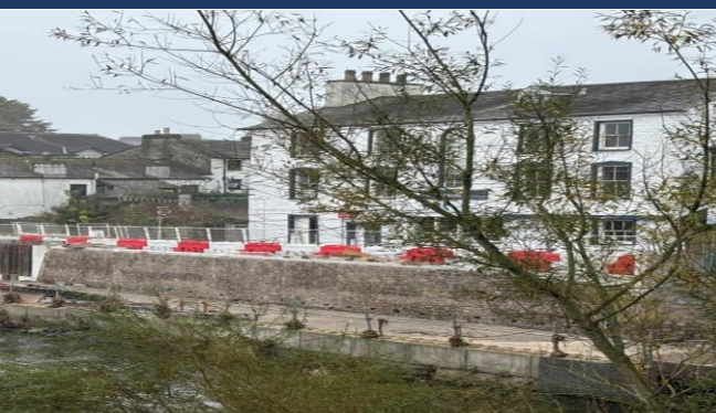
Cladded wall at Riverside Cafe
