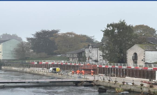
Working Platform view from Edgecombe Court
