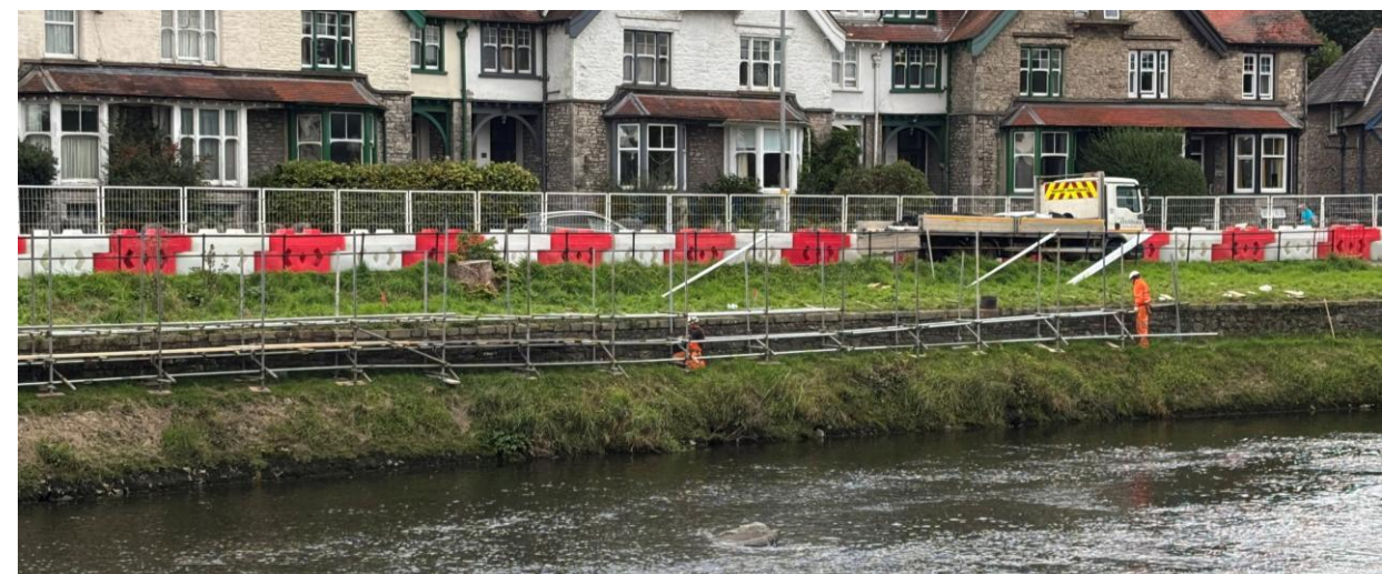
Scaffolding erection along Aynam Road
