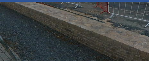
Section of flood wall cladded in natural stone
