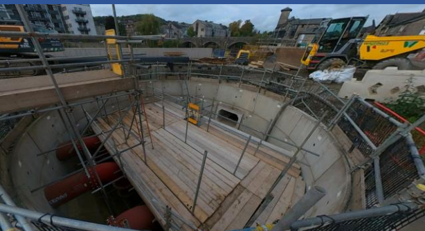
View of works inside the Wet Well
