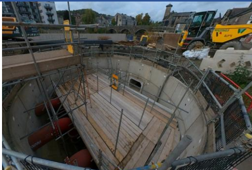
View of works inside the Wet Well
