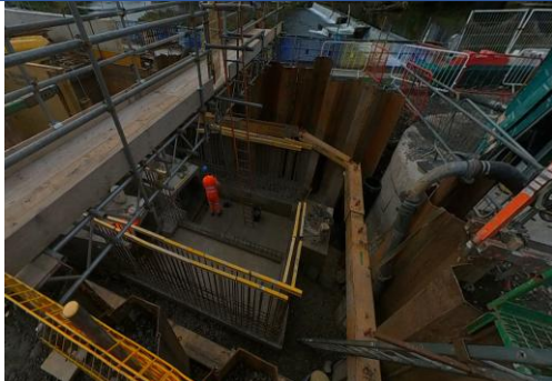
View of works inside the Overflow Chamber
