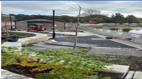
MCC and garden nearing completion
