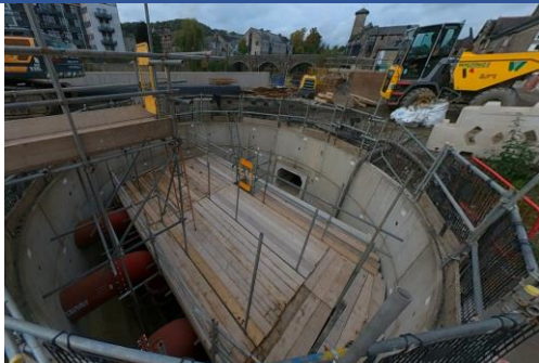
View of works inside the Wet Well
