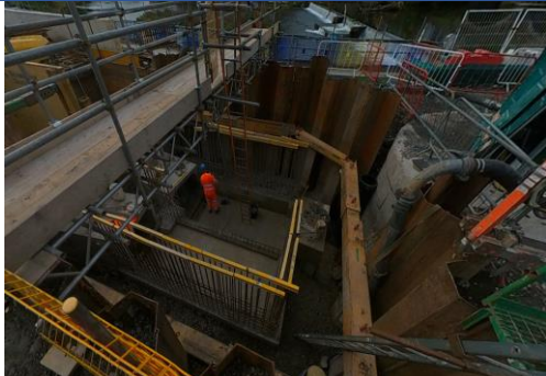
View of works inside the Overflow Chamber
