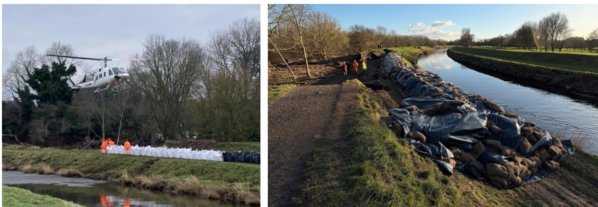
Emergency works completed at Ford Lane (Didsbury Sports Ground)
