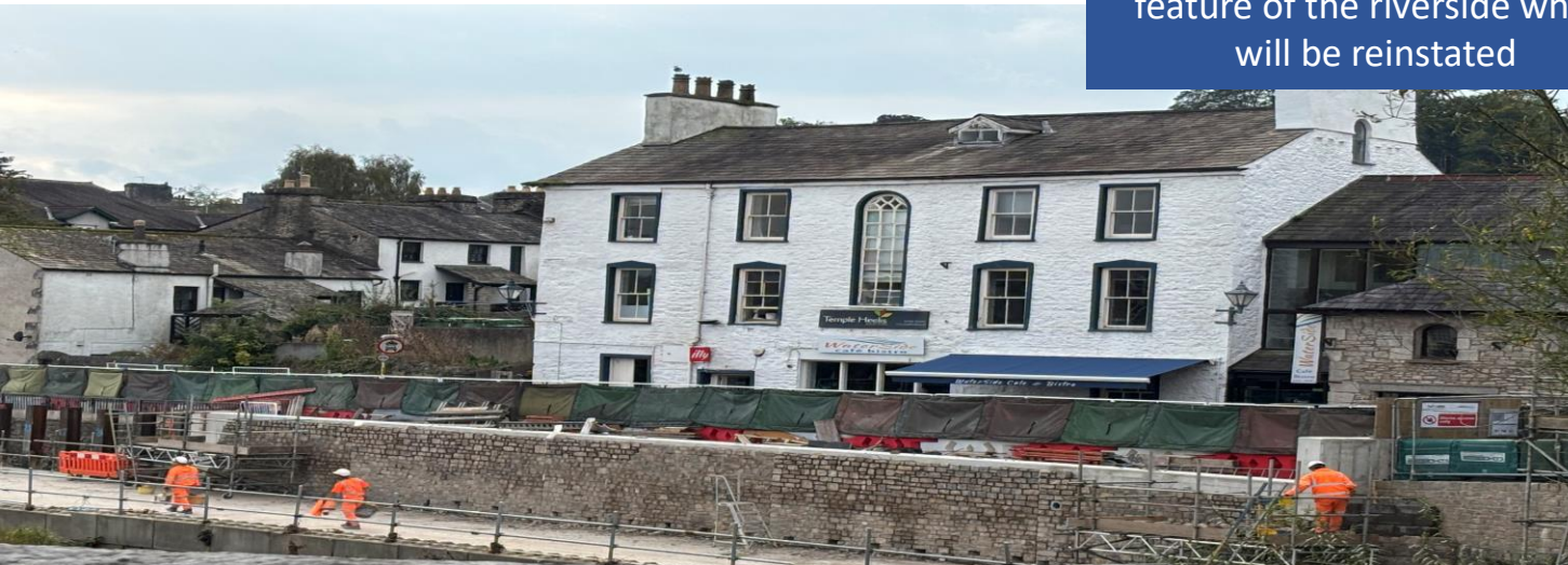
Waterside working platform showing the new concrete flood defence wall being clad – the king posts being inserted downstream prepare for the final stages of the flood wall construction.
