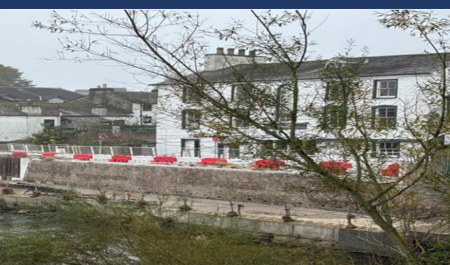
Cladded wall at Riverside Cafe
