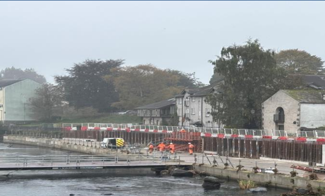
Working Platform view from Edgecombe Court
