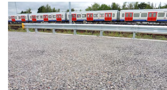
SUDS approved pavement/car park reinforcement for flood-prone areas – made from recycled plastic (British Recycled Plastic/Low Carbon Products Ltd).
