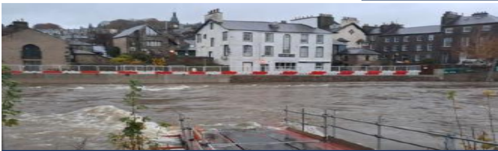
Flooded temporary bridge and working platform
