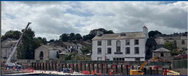
Insertion of king posts at Riverside Cafe
