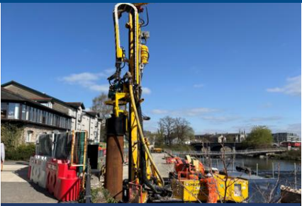
Piling at Edgecombe Court
