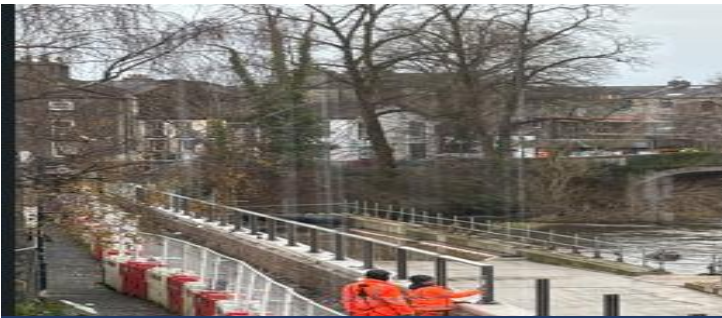
Installation of the glass panels
