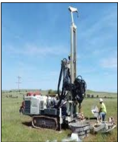
Sonic drilling rig
