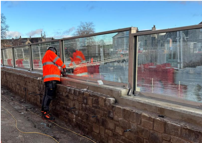
Finishing touches to the flood defence glass panels along Waterside
