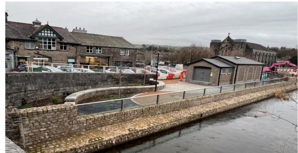
The Fern Garden and Motor Control Centre showing glass panels along the flood wall.
