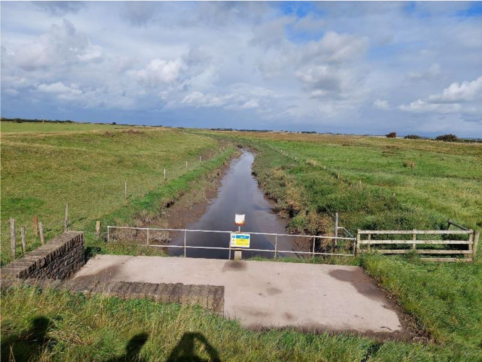
Cocker channel looking downstream from Cocker Bridge sluice gates
