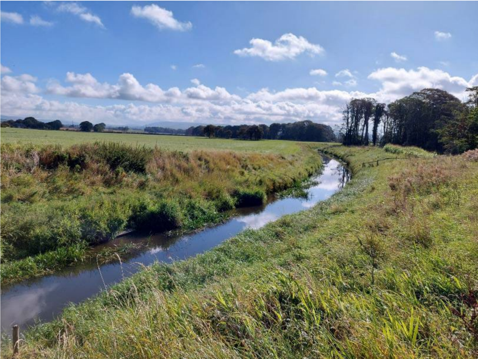
Cocker channel looking upstream from Cocker Bridge sluice gates
