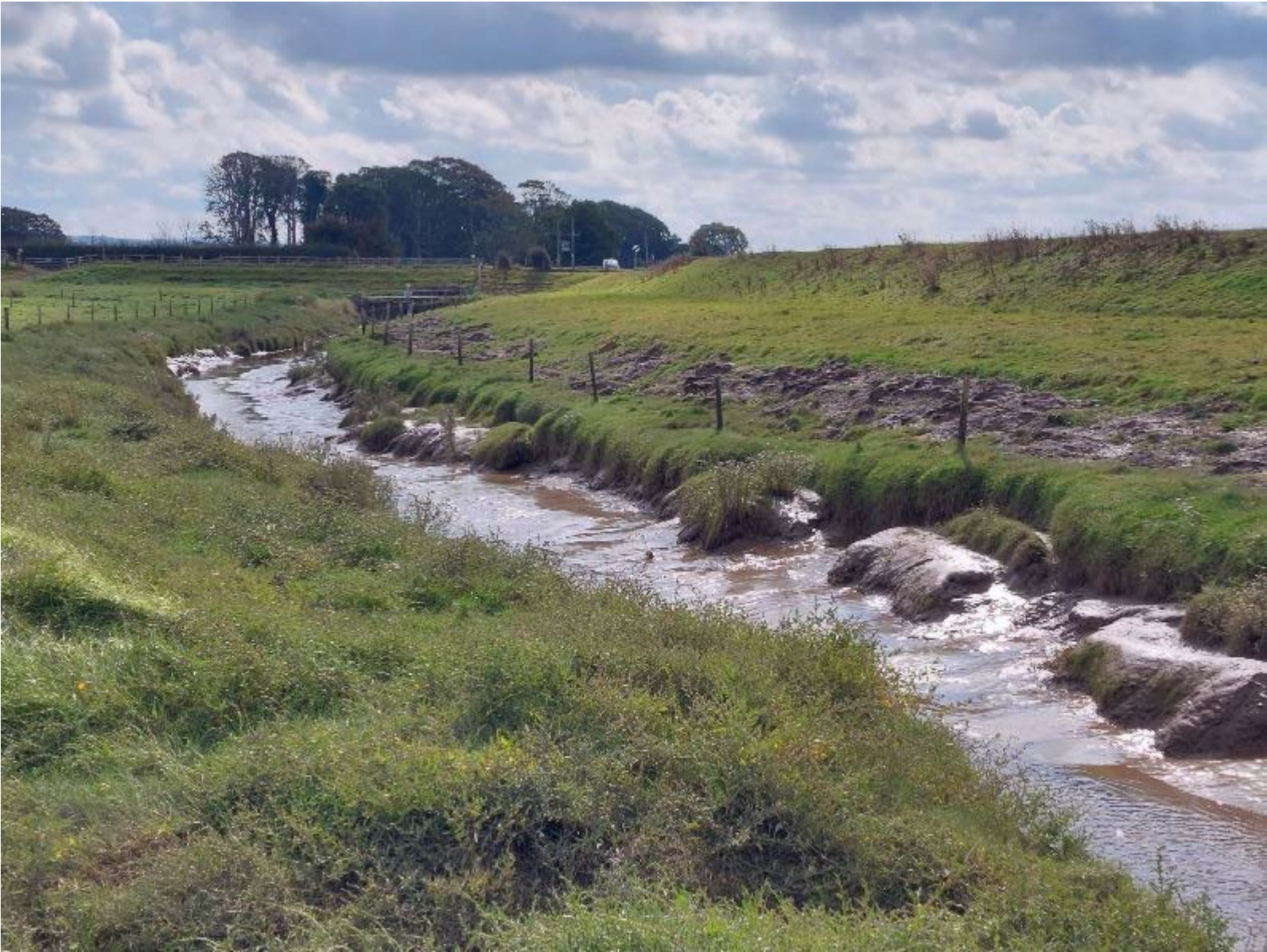
Cocker Tidal Channel – ‘new’ cut reach slightly further downstream from Cocker Bridge sluice gates
