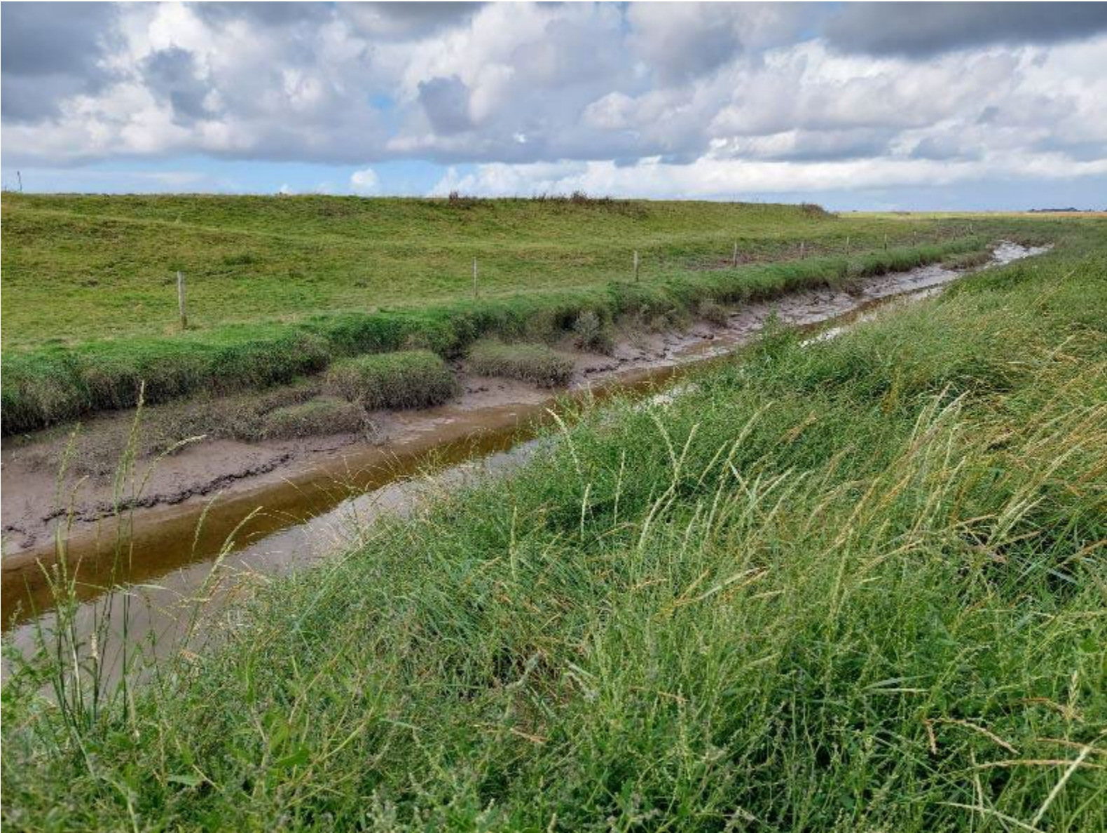
Cocker Tidal Channel – ‘new’ cut reach immediately downstream from Cocker Bridge sluice gates
