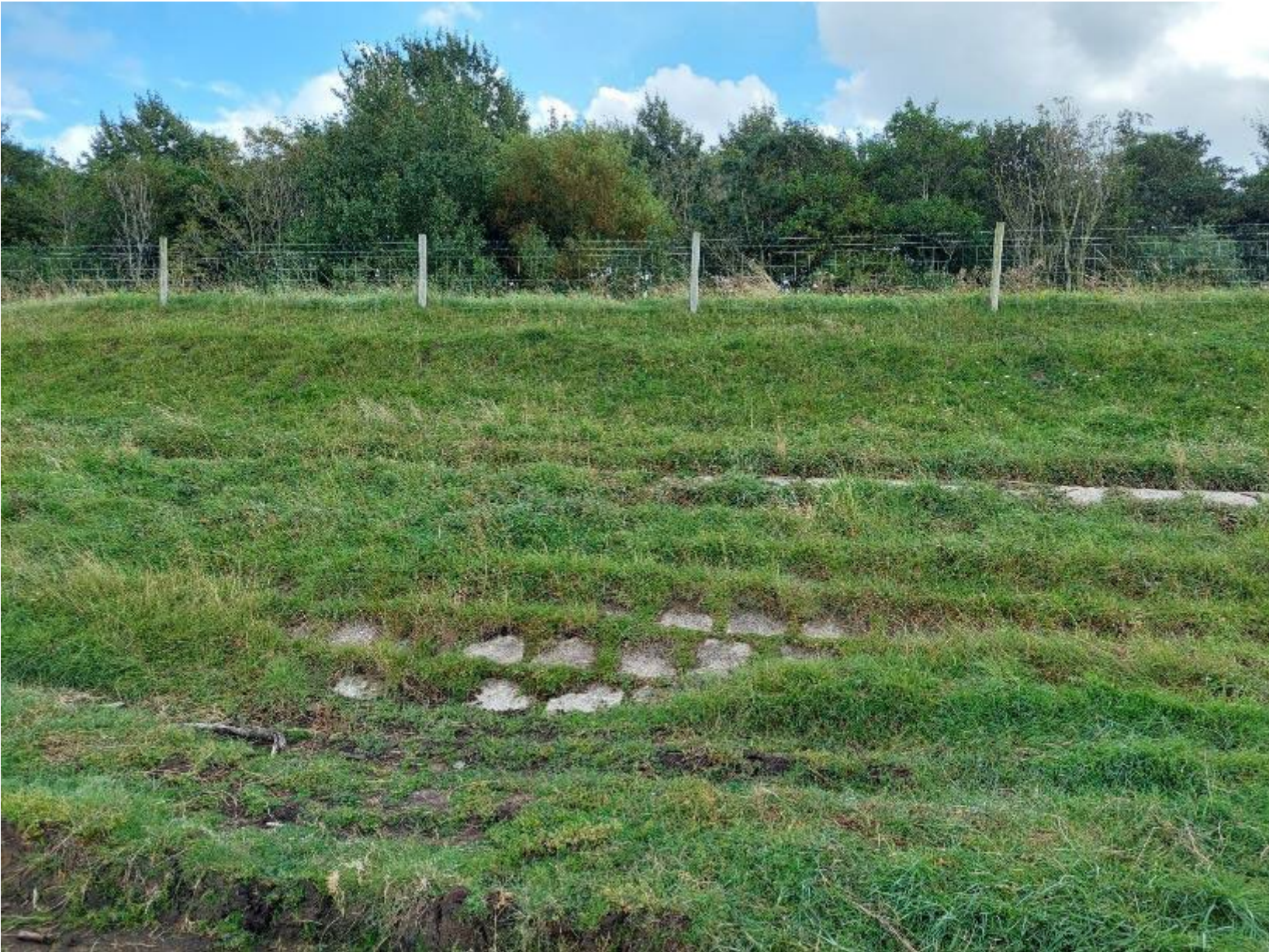
Flood embankment between Cocker Bridge and Patty's Farm
