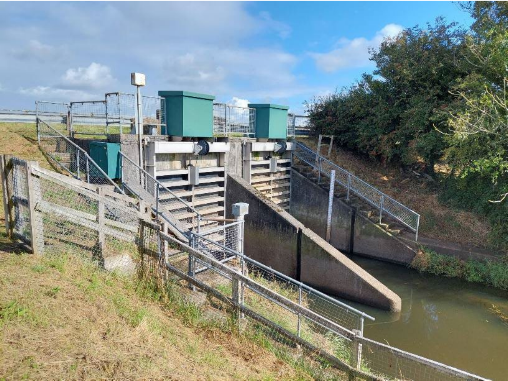
Cocker Bridge sluice gates – upstream side
