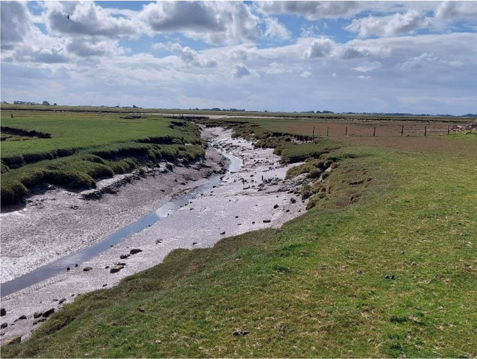
Intersection between Cut and Natural Channel from Bank End Tidal Flap
