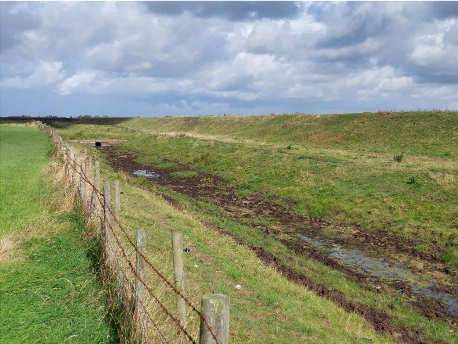
Cockerham Marsh SSSI –view of Delph ditch and flood embankment
