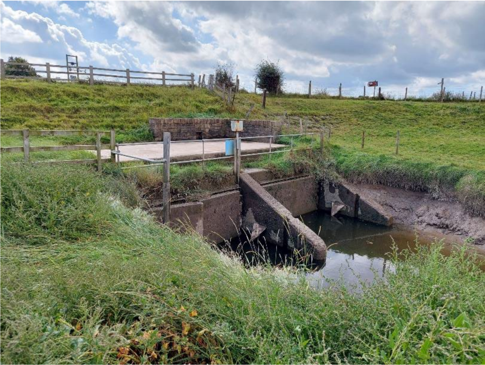
Cocker Bridge sluice gates – upstream side
