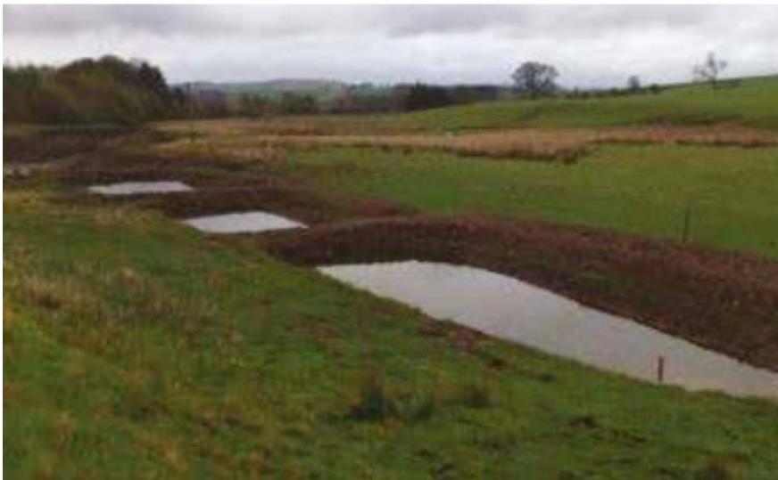
Figure 23. Three sediment traps constructed in series to intercept surface runoff and encourage settling out of sediment in the River Coquet catchment, Northumberland (© Nick Barber, Newcastle University).
