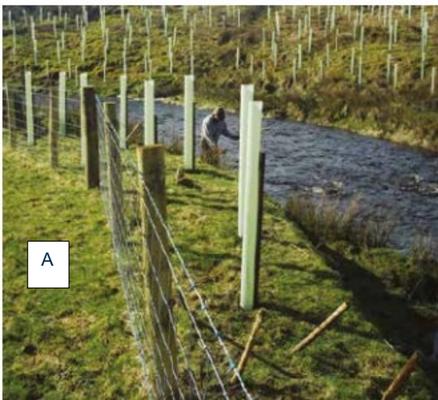
Figure 15. Fencing stabilises riverbank and reduces sediment loading in stream
