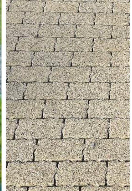
Granite finish - concrete block permeable paving
