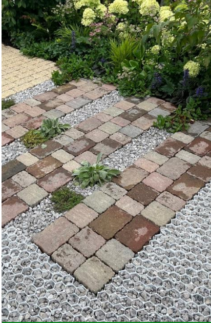
Gravel grids and permeable block pavers
