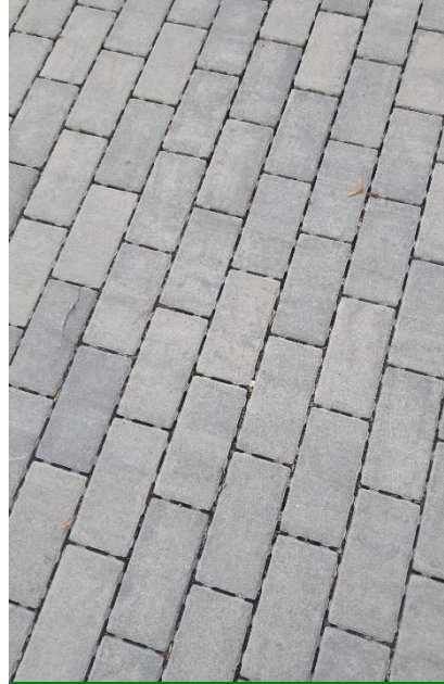
Concrete block permeable paving
