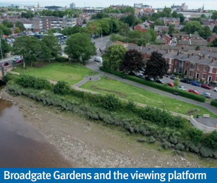
Broadgate Gardens and the viewing platform
