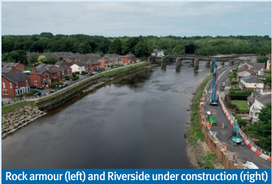
Rock armour (left) and Riverside under construction (right)
