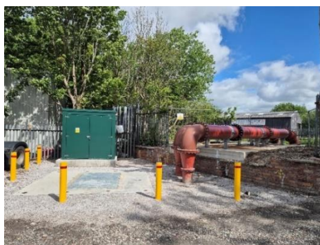
Liverpool Road Pumping Station
