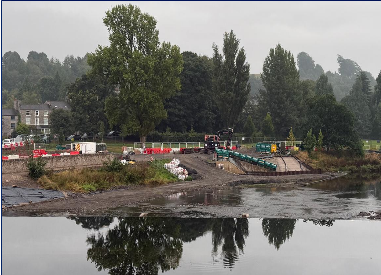
Picture showing gravel removal and out fall works near completion
