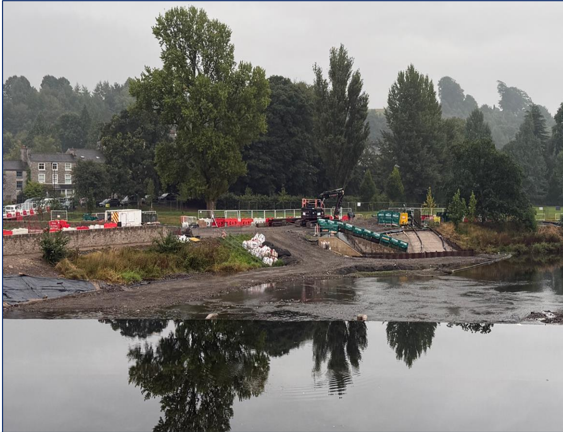
Picture showing gravel removal and outfall works area
