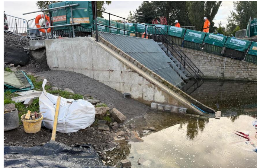
Picture showing remaining cladding to the wing wall section
