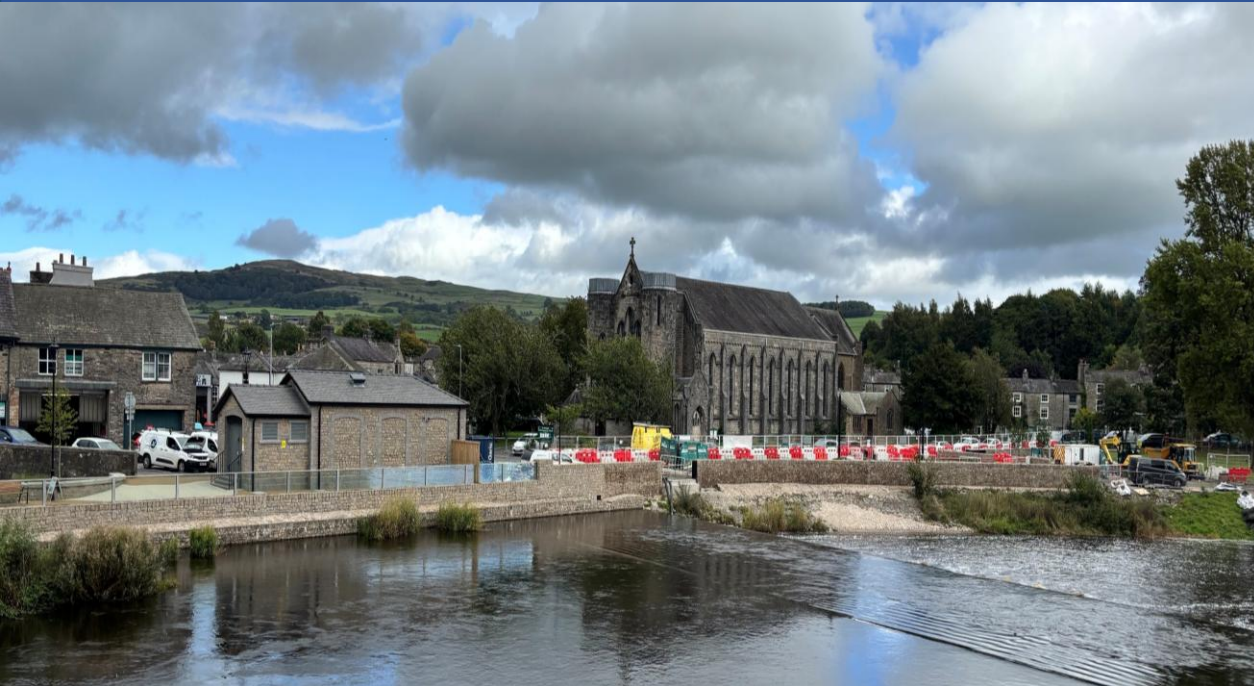
Flood defence wall near completion following the huge engineering task of the sewer and Stock Beck diversions and the construction of the 9 x 6 metre wet well under ground
