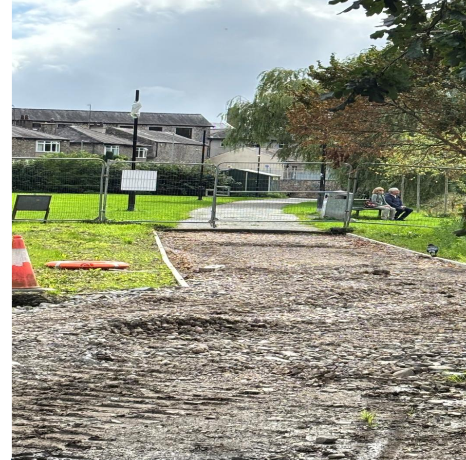
The re-instatement works continue replacing kerb stones ready for the path to be prepared and tarmacked
