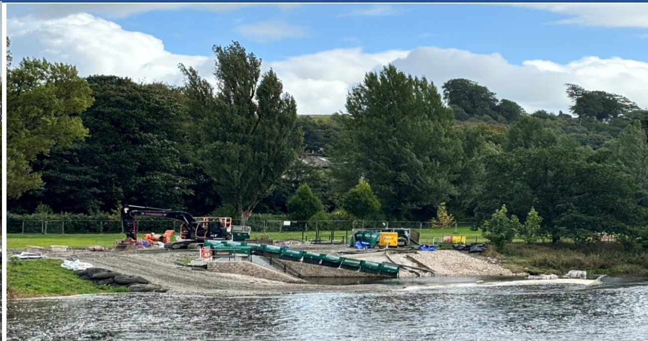
The stone cladding on the outfall and revetment is progressing and working up the banked area
