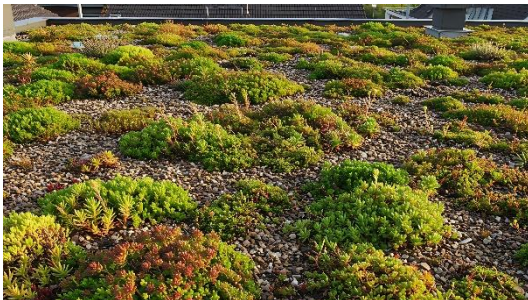
Sedum and gravel roof
