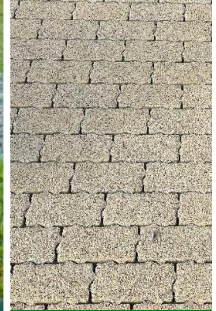
Concrete block permeable paving Unpave the Way Garden
