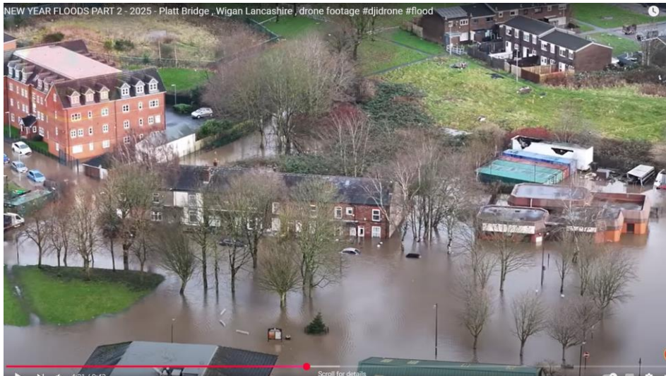
Figure 1 Platt Bridge Flooding New Year's Day 2025
